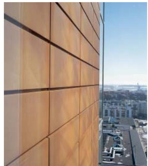
Cor-Ten steel, which was awarded the steel structure prize in 2000, has been used in both the frame and the details of the building.
