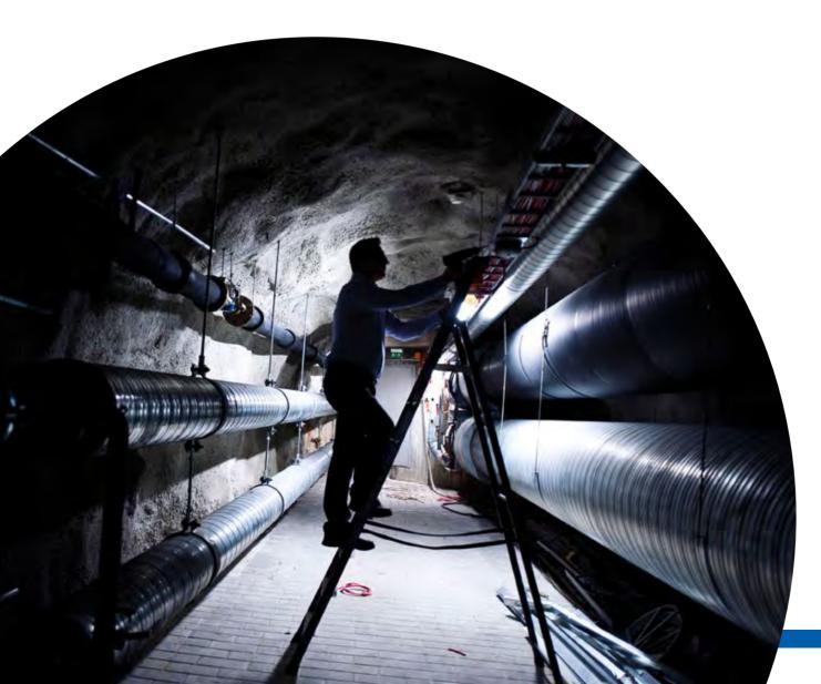
To top this, Helsinki has the world's largest heat pump that produces district heating and cooling in a single process. The unique system, situated in a rock tunnel some 25 m underground, uses both sea water and purified waste water for cooling and heating purposes. As a result, the CO<sub>2</sub> emissions of the plant are 80 percent smaller than those of an alternative production solution.
