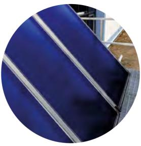
The solar thermal collectors on the roof of the complex heat the pool water in the seven pools. The collectors yield approximately 120,000 kWh of thermal energy per year, about 5 percent of the total energy needed to heat the water. The photovoltaic panels on the roof generate some 45,000 kWh of electricity annually; this covers 3 percent of the actual need.
